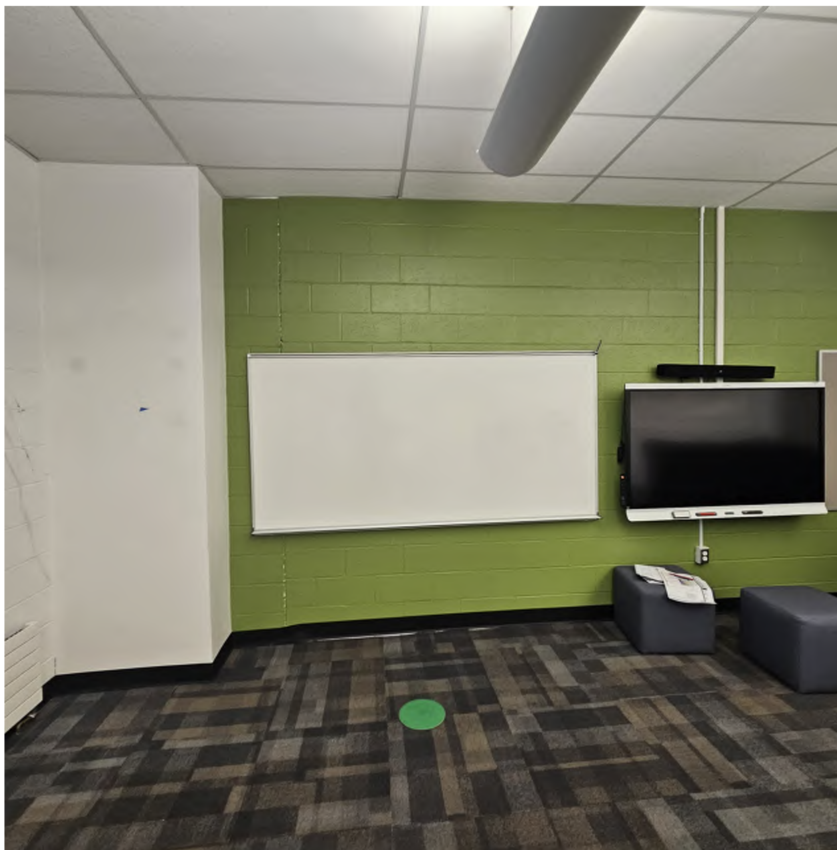
4 EXISTING MB & CAULKING JOINT G125
